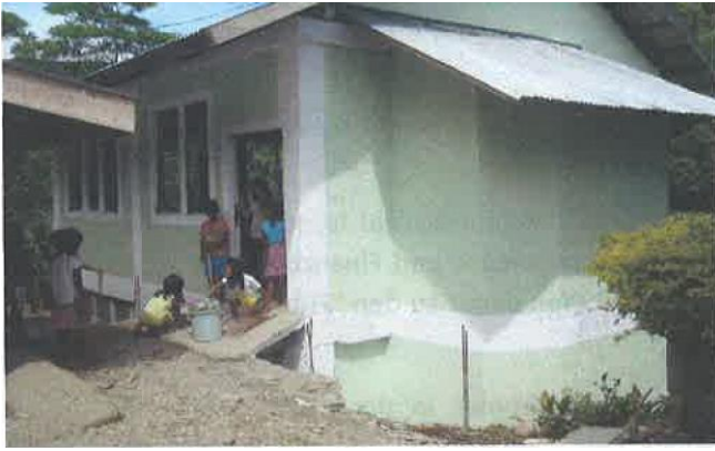
June 2019, the first school day in the new building
